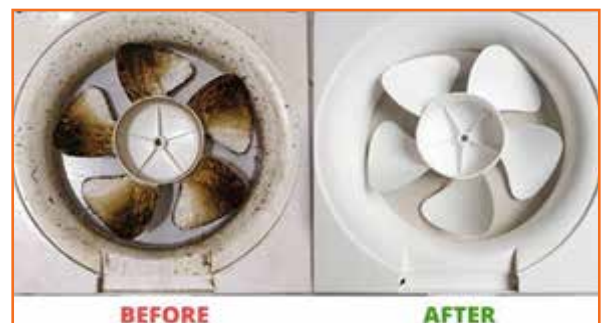
Fig.4.1.29: Cleaning Exhaust Fan
