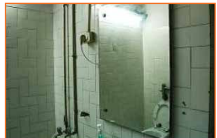
Fig.2.2.14: Cleaning of Bathroom -8
